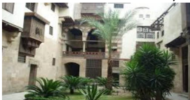
pic No. (9) indicating the internal backyard of Bayt Al-Suhaymi – Egypt
