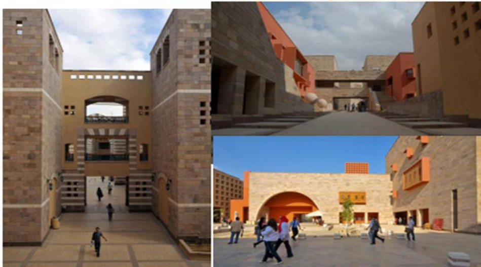
pic Nos. (29, 30, 31, 32, 33 and 34) indicating the internal and external design of the American University in Cairo, Reported by http://archnet.org/sites/6717/media_ contents/ ArchNet
